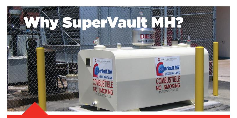
**SuperVault MH** double-wall, fire-protected aboveground storage tanks feature an inner and outer steel tank with lightweight thermal insulation that exceeds a 4-hour fire test.
