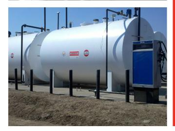
**FLAMESHIELD**® Fire-Tested aboveground storage tank is manufactured with a tight-wrap double-wall design.
