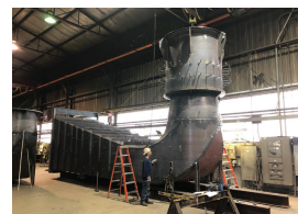
Hydro Power Draft Tube
